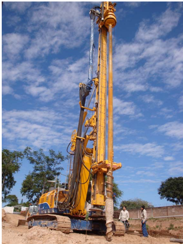
Fig. 4 The FDP pile construction unit
